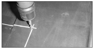
45. Using a 5/16" drill bit, drill a hole where the horizontal and vertical lines intersect.
