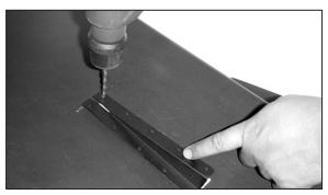
47. Hold the right angled "Z" bracket in place, using a 3/16" drill bit, drill out the five outer holes.
