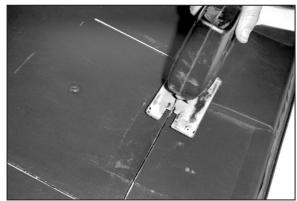
46. Using a jigsaw, cut along the horizontal and vertical lines.
